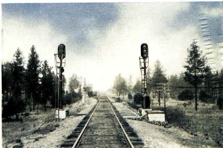
Figure 4 Type D Color-Light Signals Great Northern Railway
