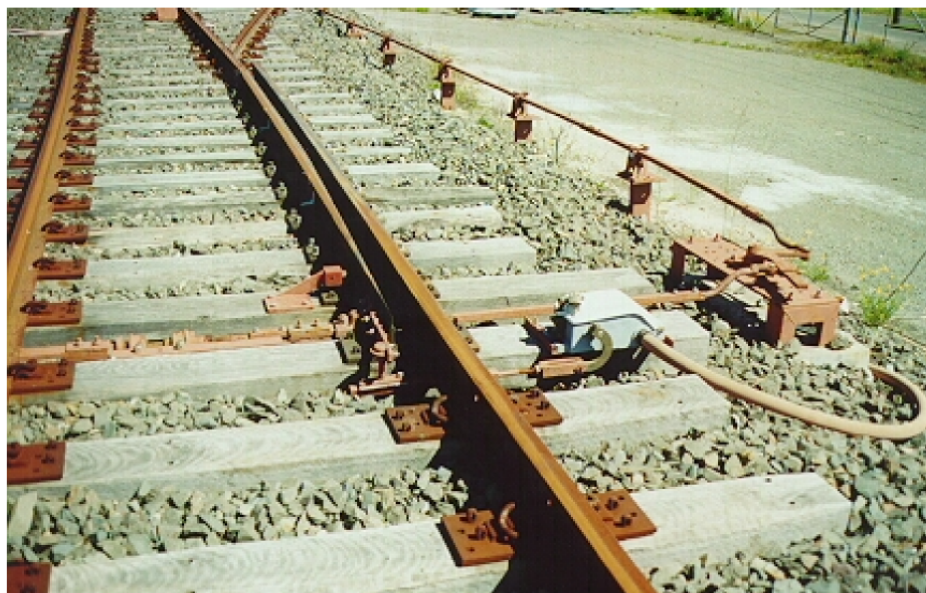
Figure 2.1.12 - Typical Catch Point
