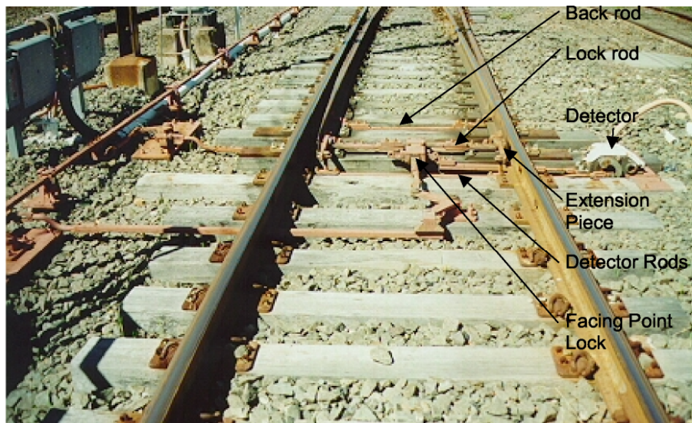
Figure 2.1.11 -Typical Facing Point
