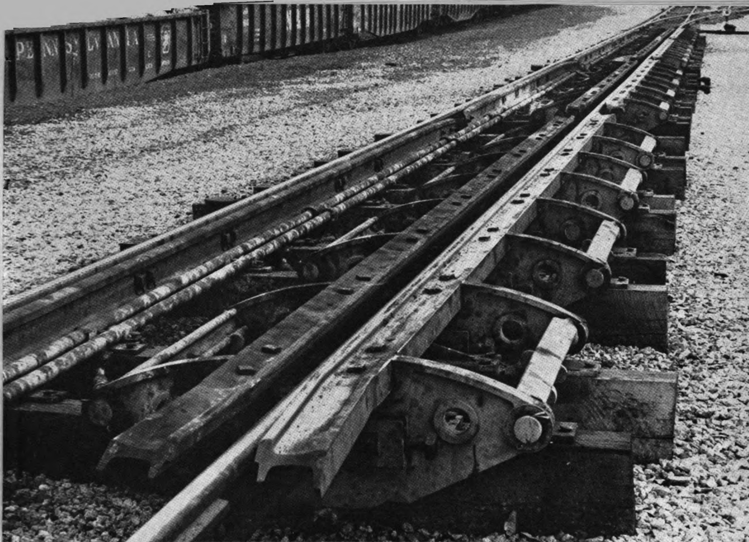
Retarders are weight-responsive in that car pressing downward increases retarding force due to mechanical linkage.
