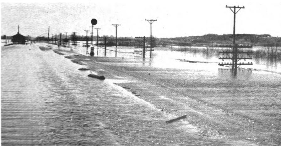
Rock Island line near Nahant, Ia., shows how pole lines may escape severe damage due to high water, unless there is a washout.
