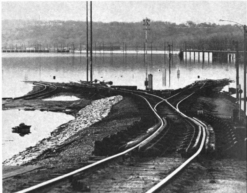
Water covered Milwaukee Road's St. Paul, Minn., classification yard to a depth of about 8 ft. This is view from hump looking northward.
