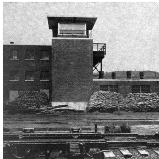
Retarder tower was sandbagged to prevent debris from damaging building.
