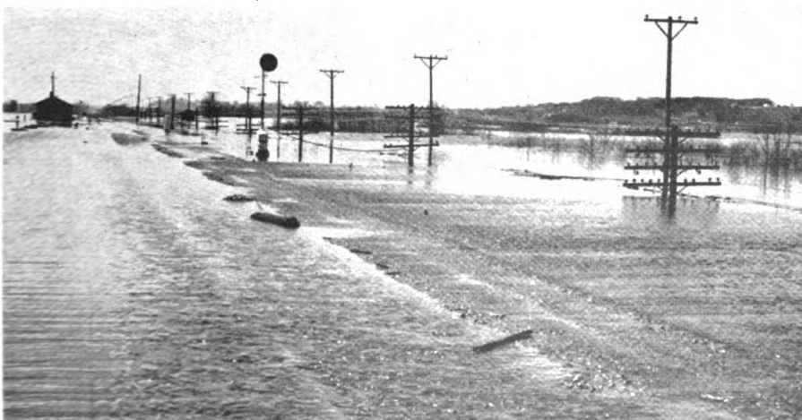
Rock Island line near Nahant, Ia., shows how pole lines may escape severe damage due to high water, unless there is a washout.
