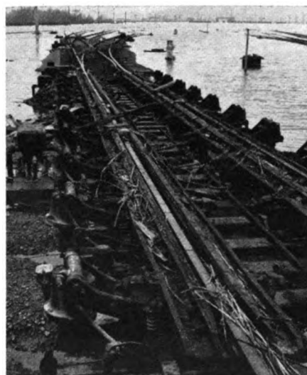
After water receded from retarders debris remained to be cleaned out.
