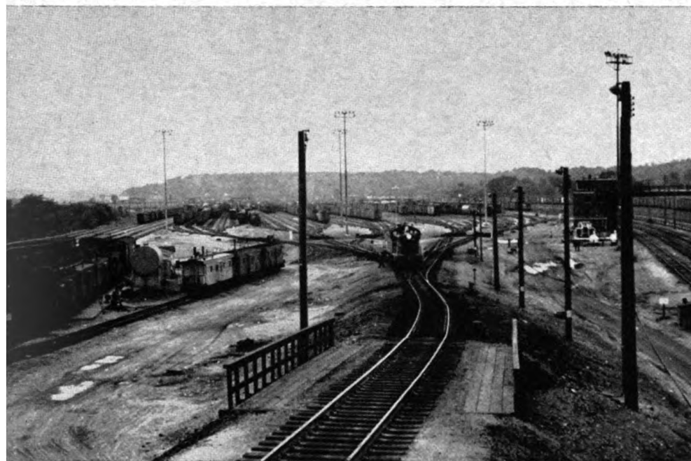
When restoring MILW yard to service, switch engine was run over class tracks several times to wear off rust and restore shunting sensitivity.
