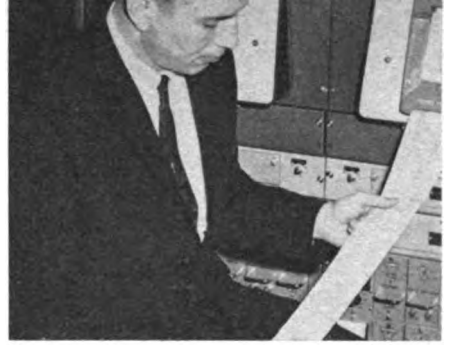
Hotbox detector recorders are in the Perry, Iowa dispatcher's office.
