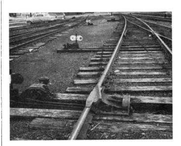
When you see a Hayes Model HB Derail in "open" position (on the rail) its purpose is immediately apparent: it commands all traffic to stop at that point. Disobedience of this order brings instant derailment and a quick halt to further movement.
