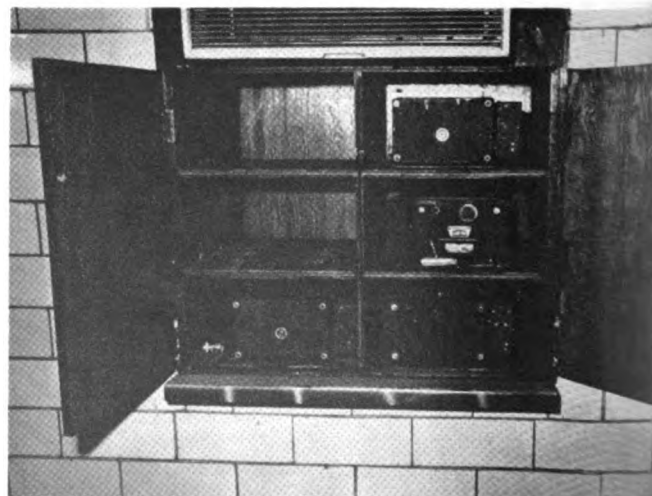
On the radio shop side of the wall cabinet, the radio unit with the handle showing indicates it is in for repair.
