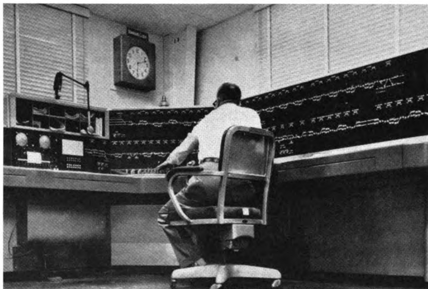
Union Traffic Control Center (Westinghouse Air Brake Co.)
