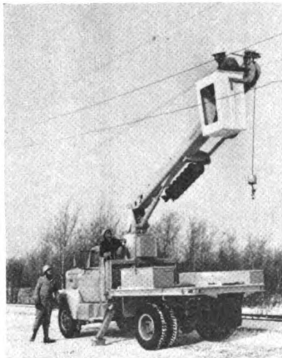
Digger-derrick digs pole holes in 3-4 minutes.
