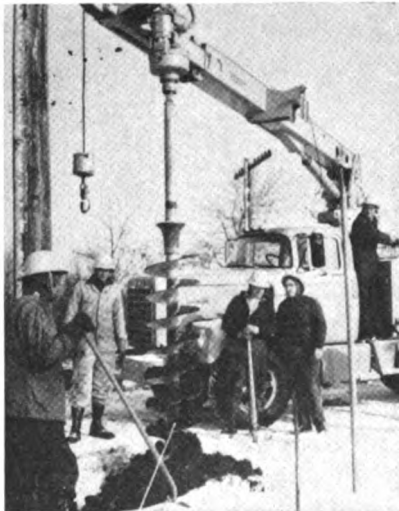
Digger-derrick digs pole holes in 3-4 minutes.
