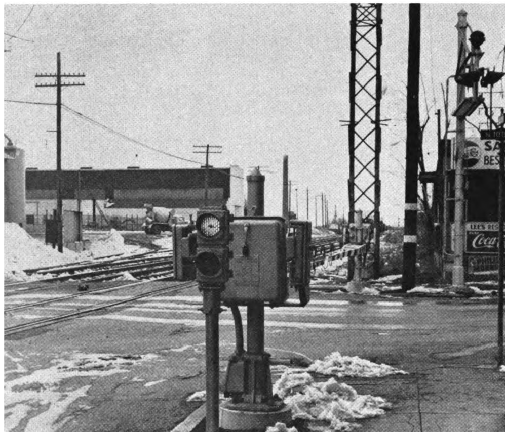
The two red lights flash alternately to warn pedestrians. Signal is used in the four blocks between 8th and 10th streets where sidewalks line both sides of tracks. Roadway gates are used on both sides of street here at 10th St because of one way traffic.
