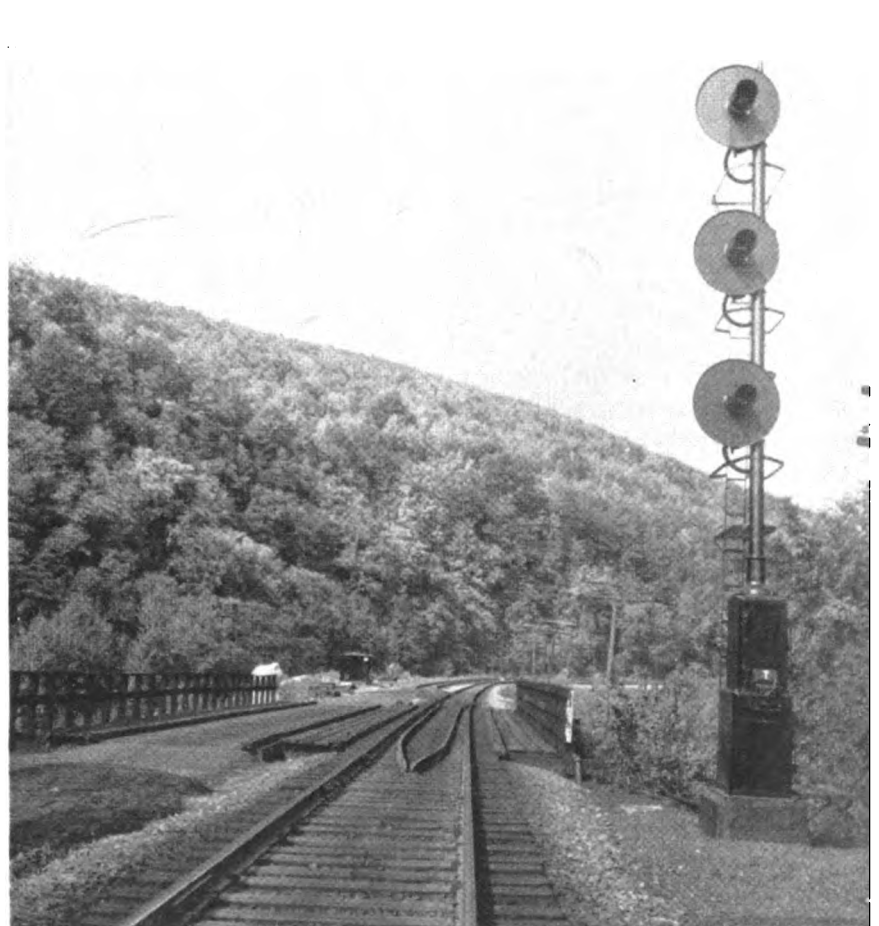
When track is removed, roadway can be built for M/W use.
