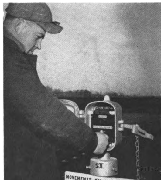
Above: Test switch is pulled down daily to check protection operation. Emergency switch is used to raise gates and cutout flashers if they operate because of a faulty track circuit or other failure.
