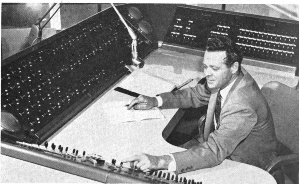
Yardmaster has keys for paging and talk-back speaker systems, radio and a dial for telephone calls. Panel at left indicates number of cars in classification tracks.
