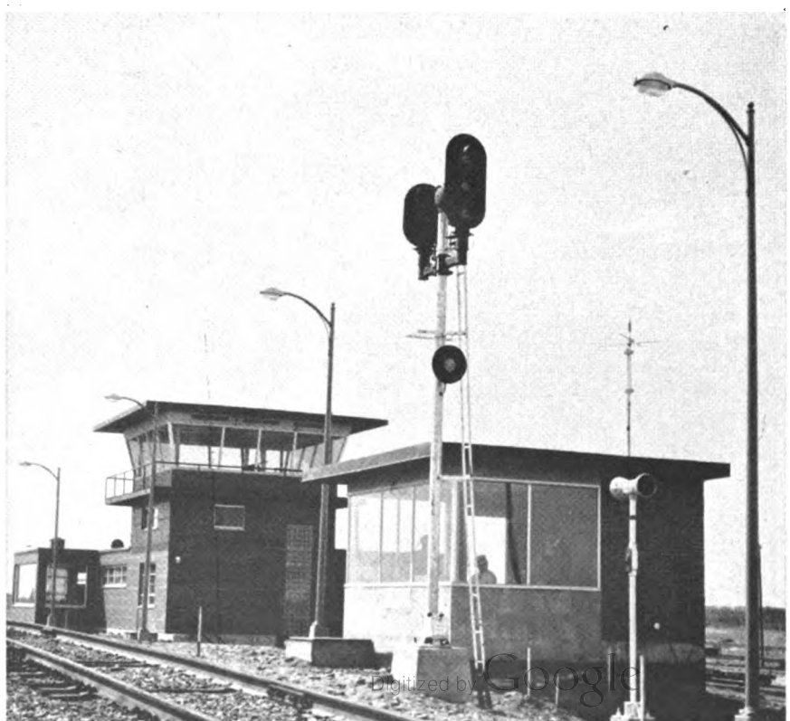
View approaching the hump with hump conductor's office in foreground and main yard office beyond. Hump conductor has automatic switching to route cars.
