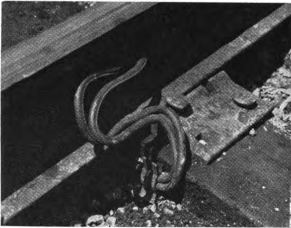
Single-conductor Number 9 cables extend from the instrument house to each rail connection.
