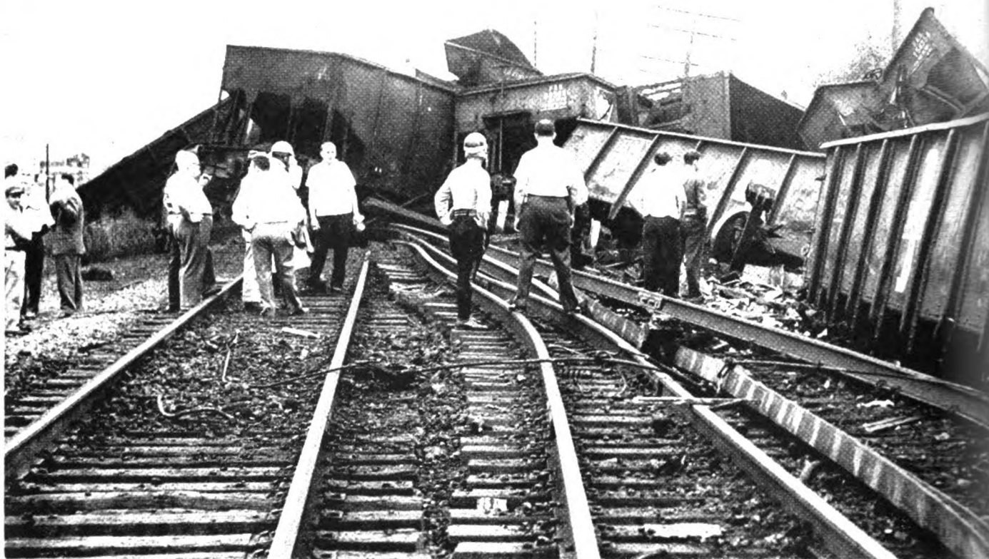
Savings on wrecks that don't happen cannot be ignored. Here, a hot box detector would have saved its cost several times over.
