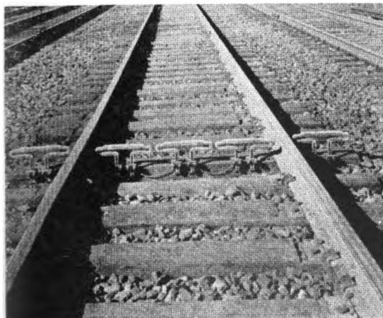
Dragging equipment breaks cast iron detector circuit.
