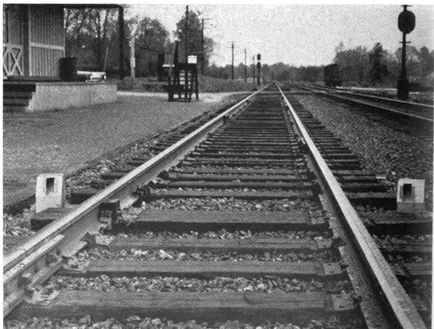
Many roads are appreciating the worth of these hot box detectors. Wrecks cost much more.
