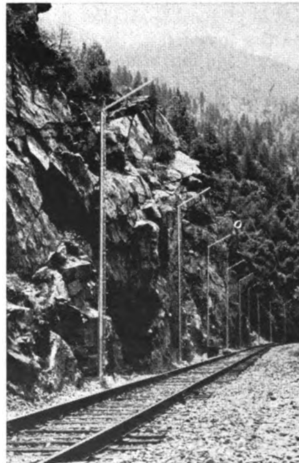
Wires form series circuit to detect rock falls.
