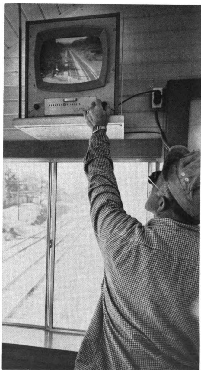
Monitor for TV camera (at Main St. at left) is in crossing tower at Mohawk St., which is 1,700 ft from the crossing.
