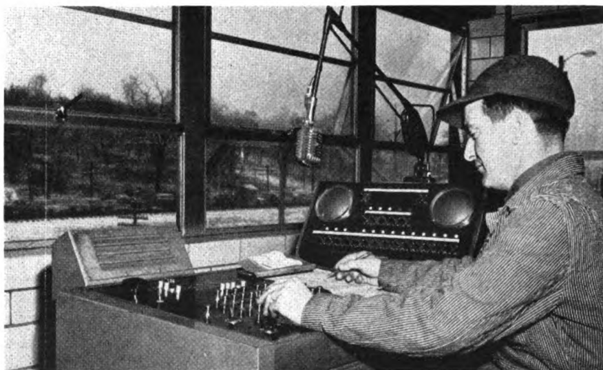
Hump conductor has radio, intercoms and talk-back speakers for communications. He punches track numbers for cuts on his automatic switching console
