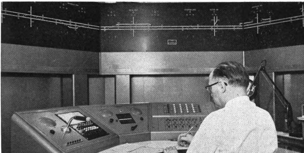
New York Central traffic control system between Toledo and Elkhart, 133 miles, is now completely in service.
