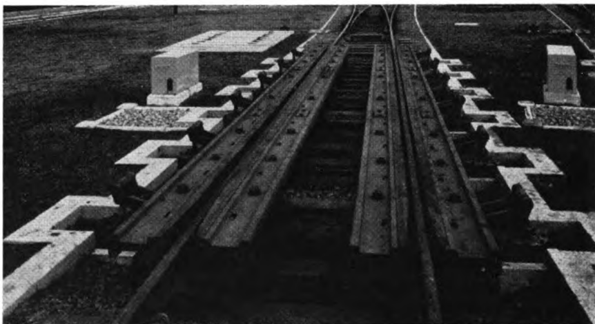
One of the secondary retarders. Radar head can be seen between the rails at the lower end. Points are also thrown by air motors.
