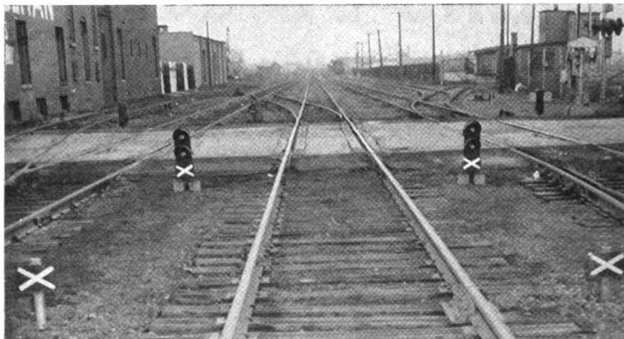
Crossing indicators on TRRASTL; limit signs in foreground
