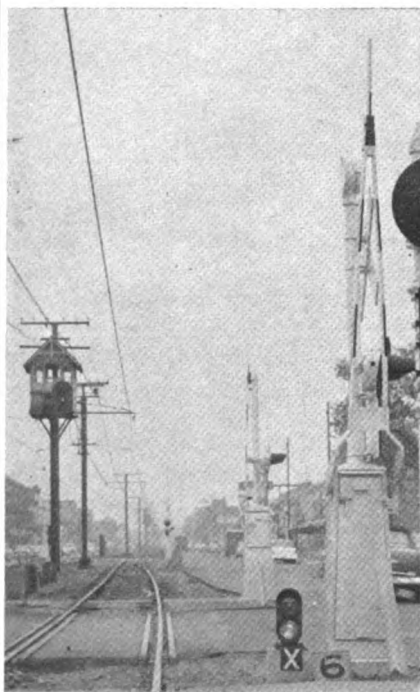
Colorlight dwarf crossing indicator in electrified territory of the IC
