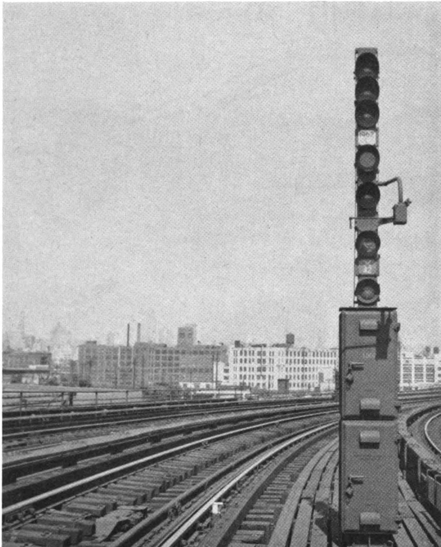
Reading from top to bottom: G, Y, R in top head of interlocking home signal are for block indications. Number plate 1962 indicates location on "C" line. "S" unit indicates signal in advance will clear on grade time control. G, R in lower head are for route indications. "X 42" indicates interlocking control lever. Call-on Y in bottom unit. Electro-pneumatic stop mechanism located between rails and trip arm at right hand side of rail. Box by middle signal head used by motorman for manual clearing of trip arm when call-on aspect is displayed
