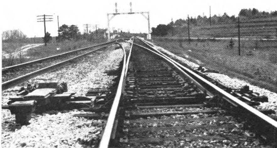
Power turnouts and crossovers are No. 20, good for 45 mph
