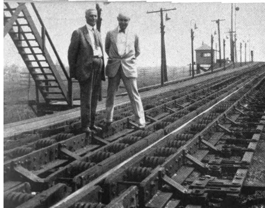
E. M. Wilcox and George Hannauer, inventors of car retarder on the IHB in 1924, standing on one of early type retarders
