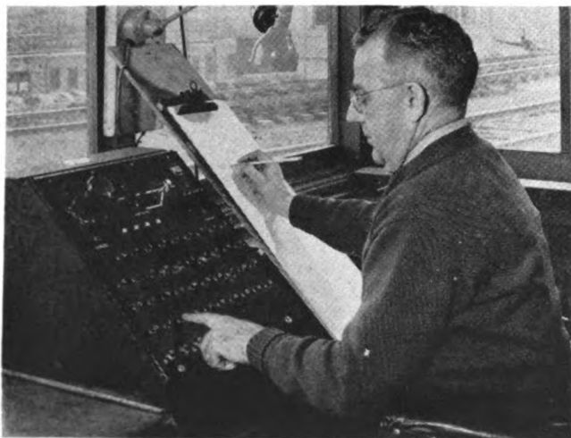
Automatic switching control, initiated by pressing button corresponding to track for car or cut, was developed in 1950
