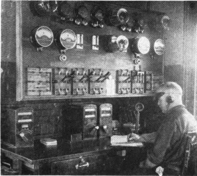
Big three-way knife switches on board controlled signals in this MP control office project in 1925
