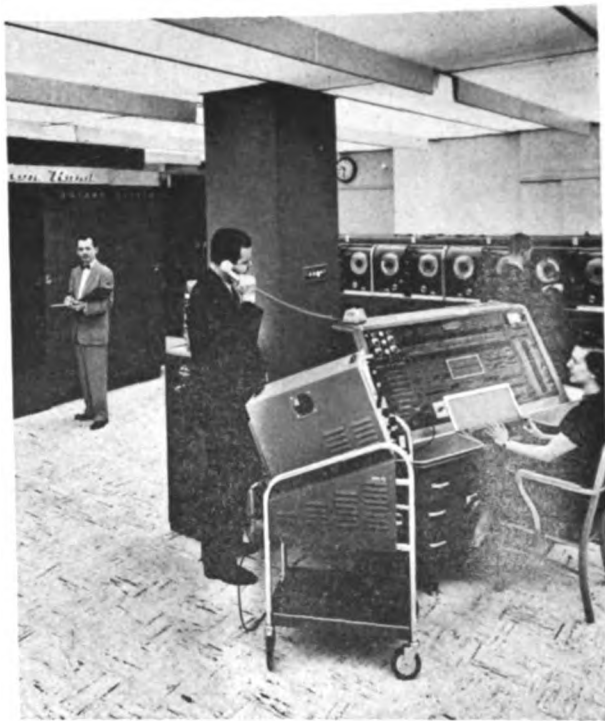
C&O's "brain" handling accounting and payroll data is fed by vast communications net utilizing printers and transceivers
