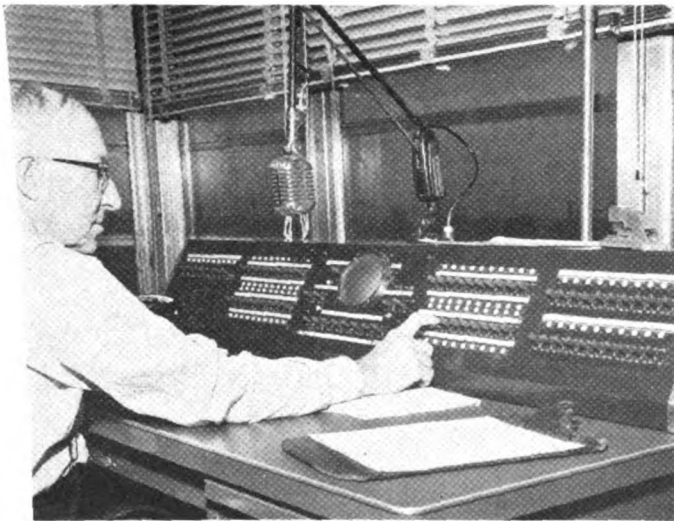
All voice circuits terminate in yardmaster's console
