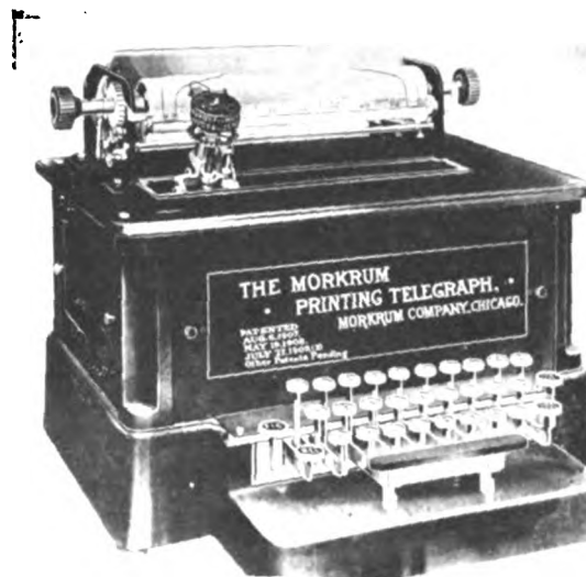
In 1910, the Chicago, Burlington & Quincy installed Morkrum printing telegraph from Chicago to Galesburg
