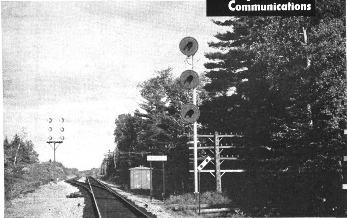
Single track with long sidings and centralized traffic control provides adequate track capacity
