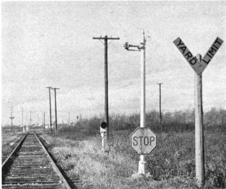
Pushbuttons and indication lamps in approach to GWWD signal
