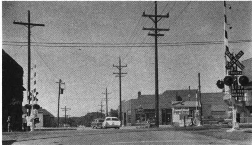
Typical crossing protection installation at Racine, Wis.
