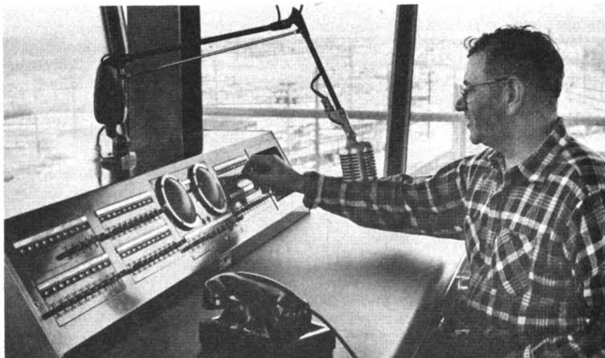
Hump yardmaster's console has voice circuits for talk-backs, pagers and radio
