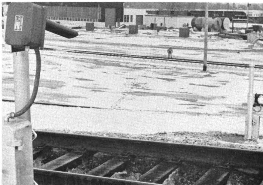
Photocells "read" cut lengths (two cells one above other) and check car location
