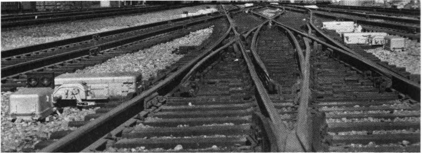
Non-interlocked power switches enable trains to arrive and depart without stopping for switches to be thrown
