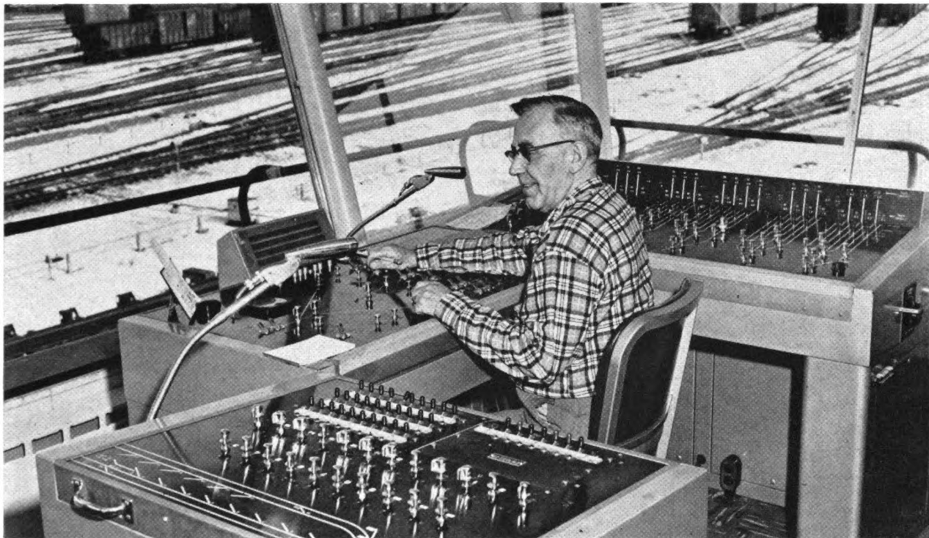
Retarder operator has control of non-interlocked switches at extreme west end of yard (panel at left foreground)
