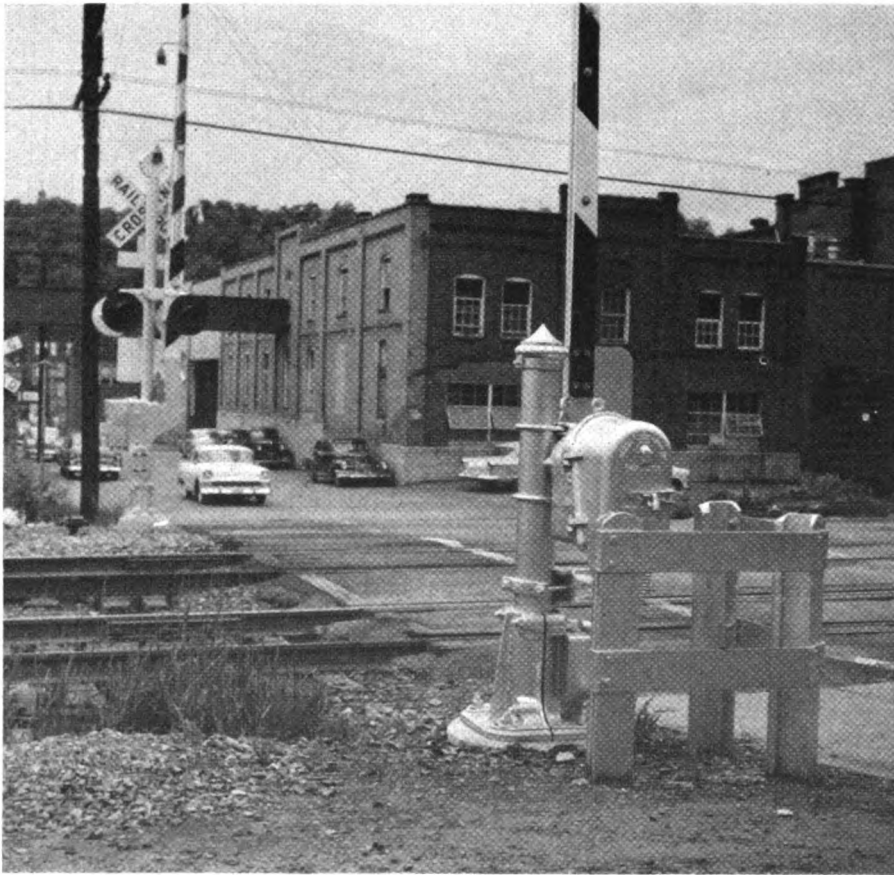
Guard for sidewalk gate is made of old rails and steel plate bolted and painted
