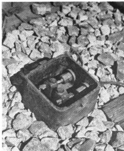
Track connections are harddrawn bronze rope-lay, through insulated bushings
