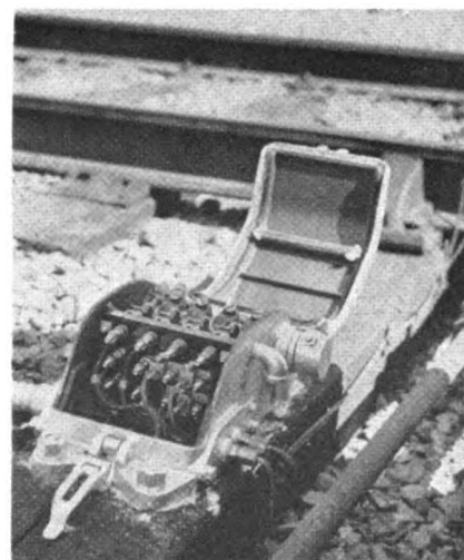
Track connections are harddrawn bronze rope-lay, through insulated bushings
