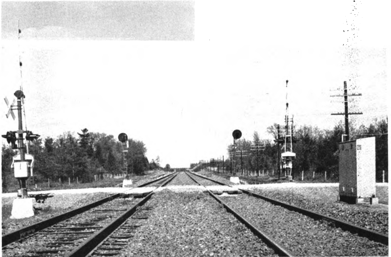
Trackwork and signaling installation work on this new mainline was performed by Canadian National forces
