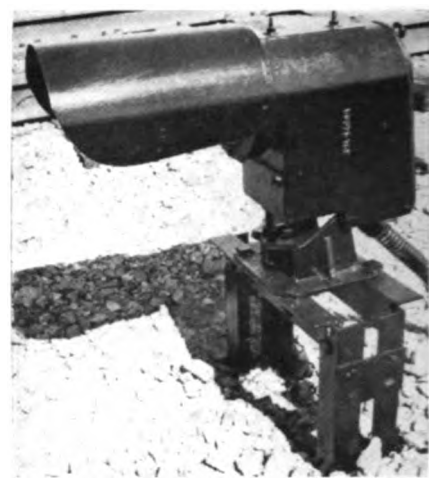
Searchlight leave-siding dwarfs on west end are on galvanized iron foundations
