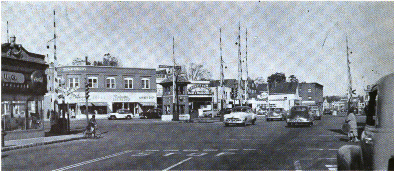
BEFORE —View of grade crossings at Church and Main streets were protected by eight manual gates
