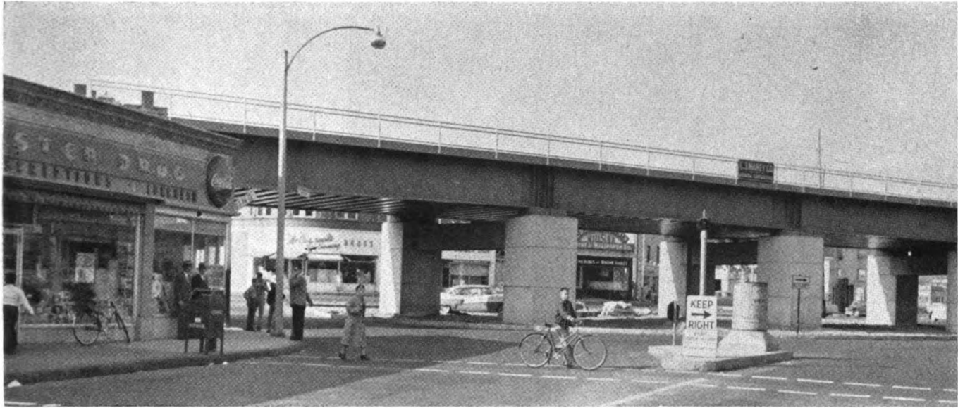
AFTER —View looking same direction showing new elevated railroad structure and streets with no gates
