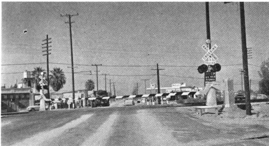
The controls for the new highway crossing gates at Niland, include special speed selections and automatic time cutouts
