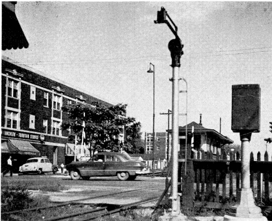
Motorman's signal and release located just short of the crossing
