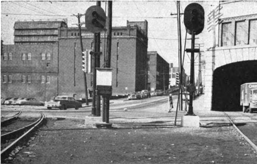
SEVENTH STREET CROSSING (looking west): signal No. 5 at right governs in both directions; additional traffic signals govern vehicular movements
