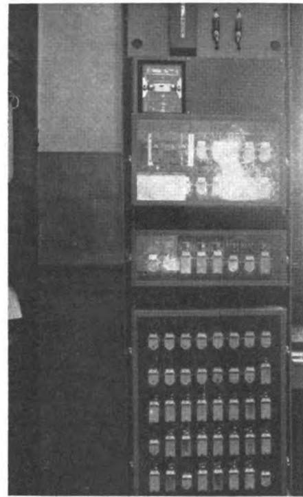
SYNCROSTEP OSCILLATOR , coding and indication relays at the control machine in the Glenwood station
