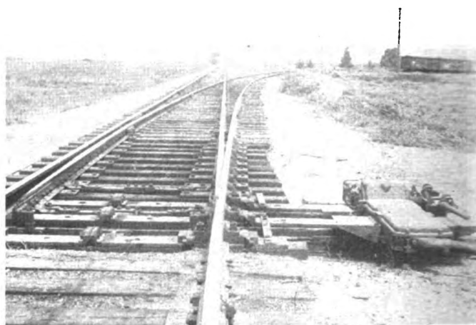
JUNCTION SWITCH for Winnipeg line. Model 5D dual-control switch machines with 24-volt heater in motor, controller compartments. Turnouts: No. 15 mainline, No. 10 yd tracks
