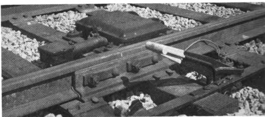
TRIP ARM RAISED to stop a train
