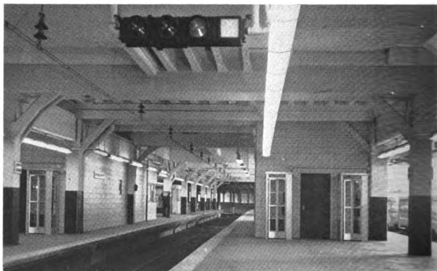
HORIZONTAL TYPE SIGNAL in Union Terminal
