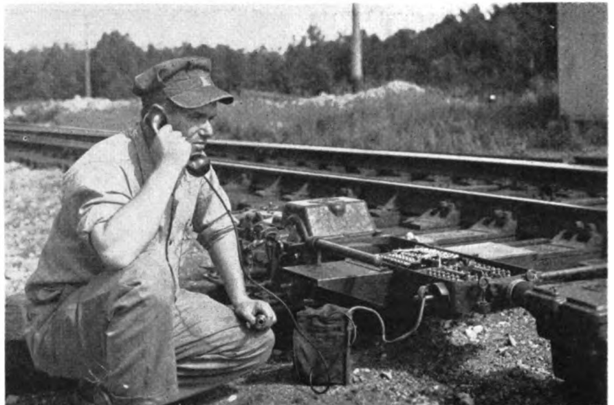
Maintainer has portable telephone that plugs in at switch machines
