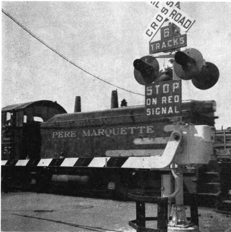
GUARDS OF OLD RAILS protect gates and signals from vehicles
