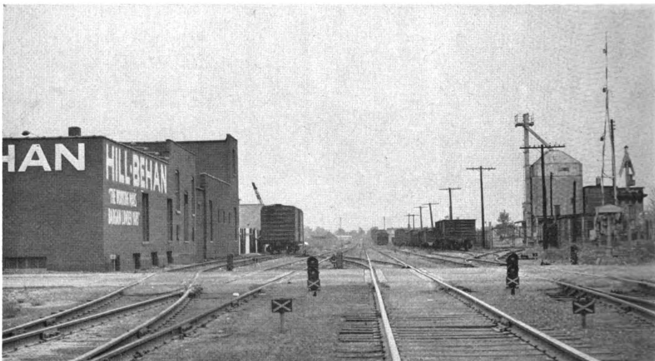
EACH CROSSING PROTECTION Indicator like a two-aspect, color-light dwarf with an "X" below it
