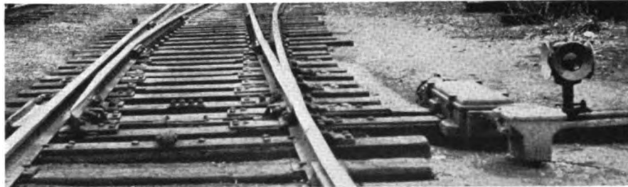
NON-INTERLOCKED POWER SWITCH machines on yard track switches
