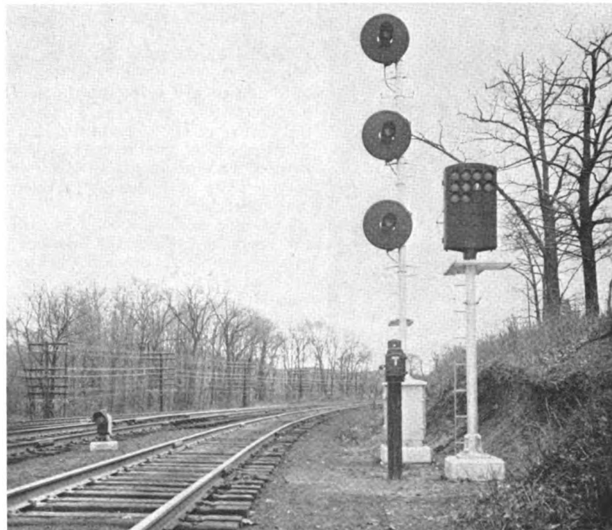
YARD TRACK INDICATOR is at right of home signal
