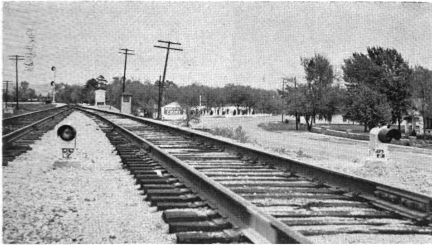
MAIN LINE DWARF saves expense of throwing siding to get clearance
