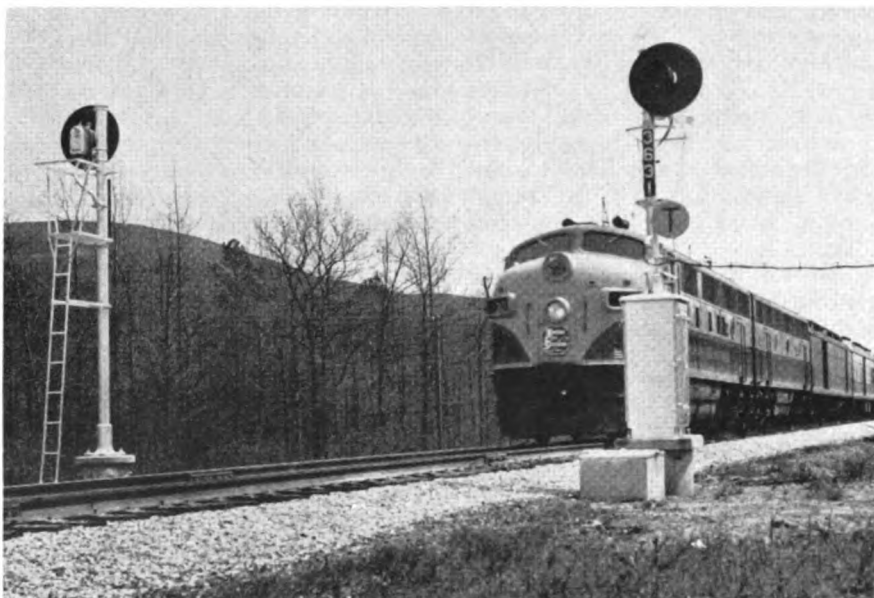
TONNAGE MARKER lets trains pass intermediate signal without stopping
