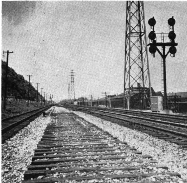
ONE TRACK WAS removed through layout at "WE"
