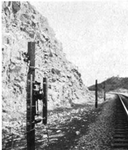
FENCE DETECTS falling rocks
