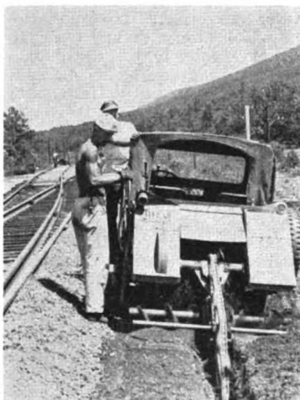
TRENCHING MACHINE mounted on a jeep
