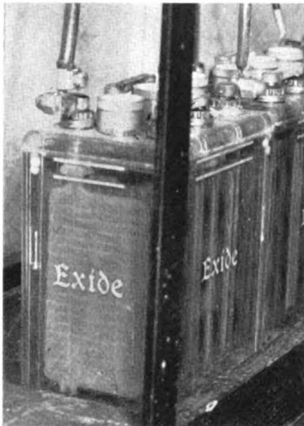
STORAGE BATTERIES for d.c. supply
