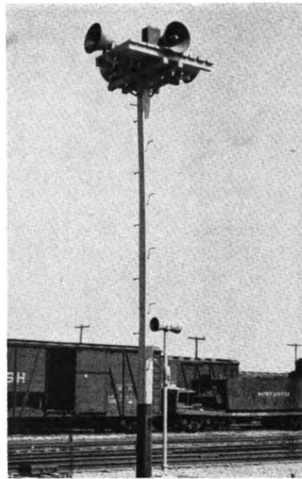
Pagers on elevated platform
