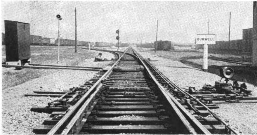
Industry track crosses main with two switches
