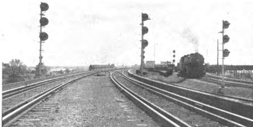
Signals 16L, 14L and 12L control trains going toward dock
